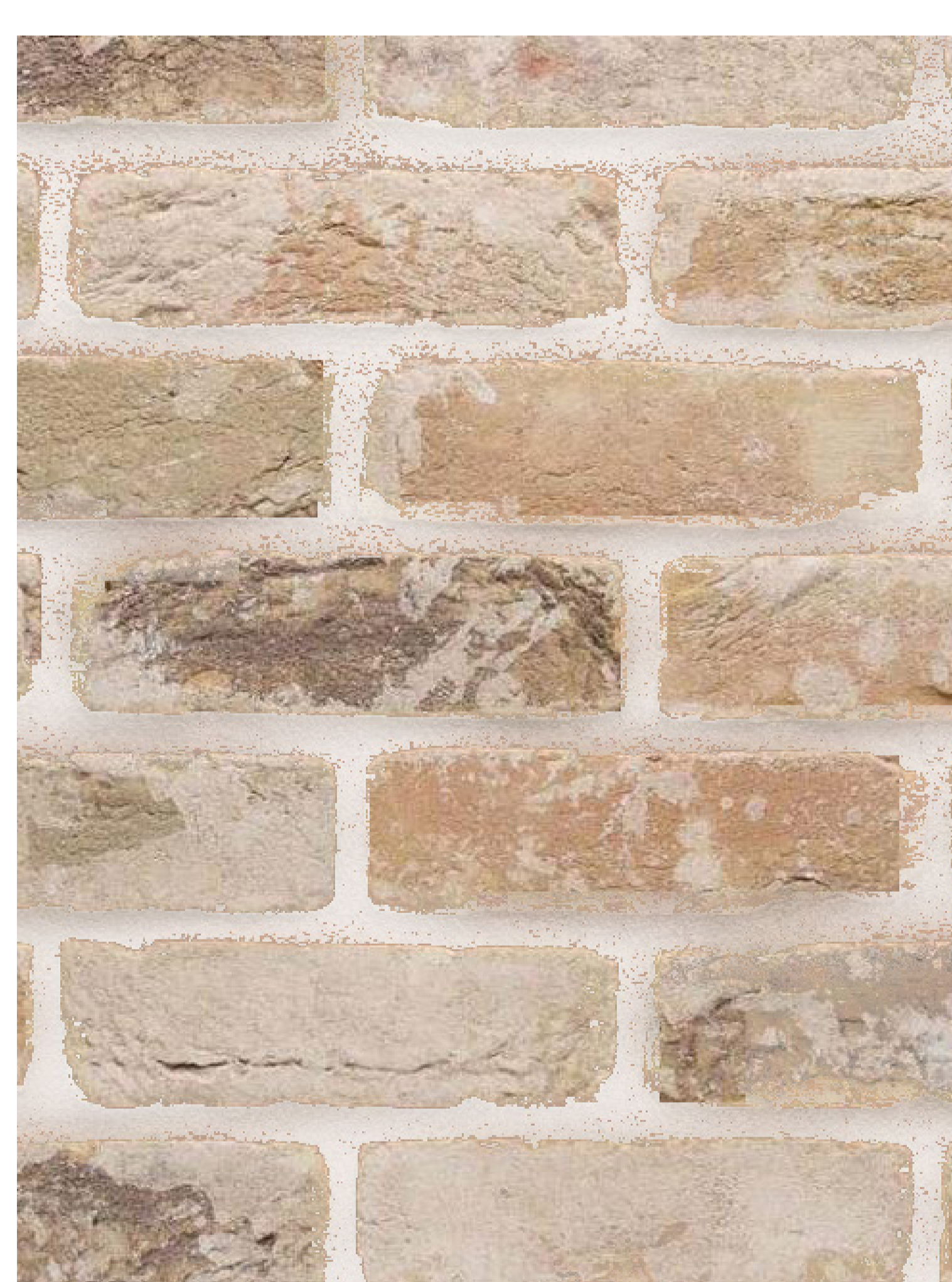
04 Light brown brickwork
