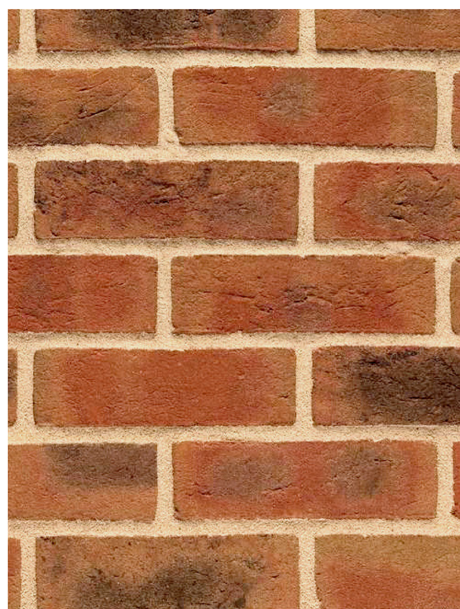
01 Red stock brickwork
